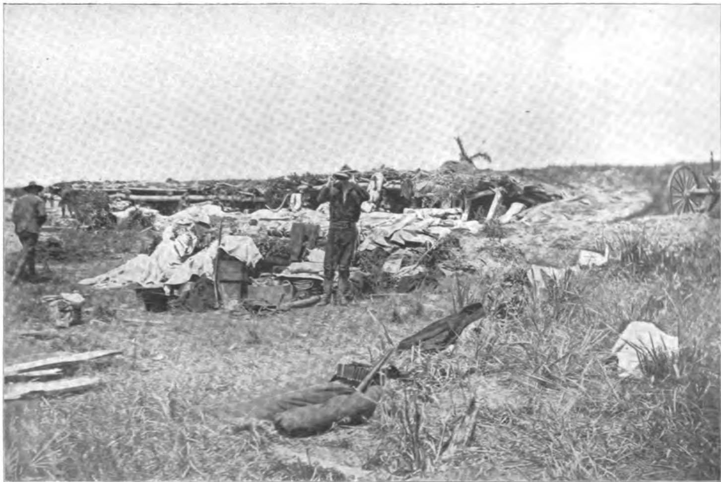
BOMBPROOFS THROWN UP BY ROUGH RIDERS TO PROTECT THEM FROM SPANISH SHELL AND SHRAPNEL.
