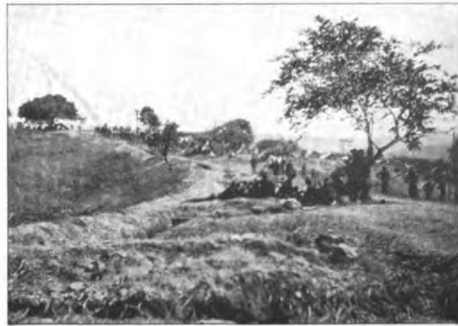
VIEW OF THE TRENCHES.
