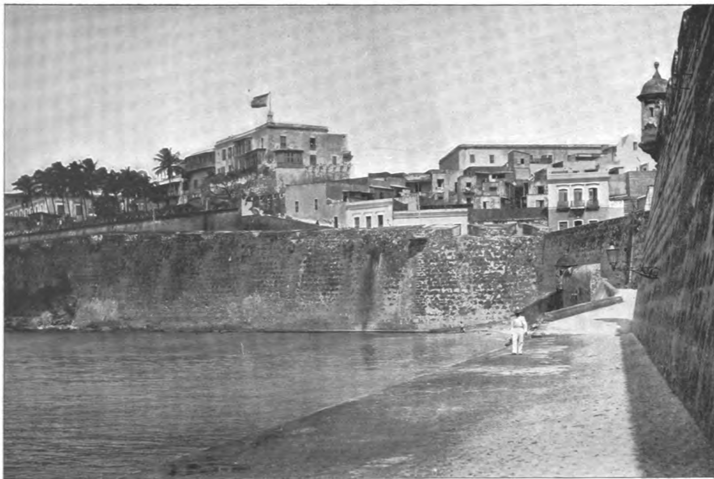
THE SEA WALL OF SAN JUAN, PORTO RICO. (Copyrighted, 1898, by J. M. Jordan.)
