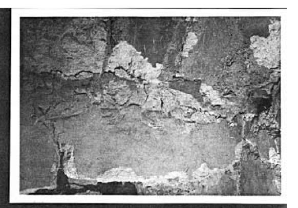
Photo 18 East wall of Bu. 196 showing dent in buckled wall seased by east wall beas.
