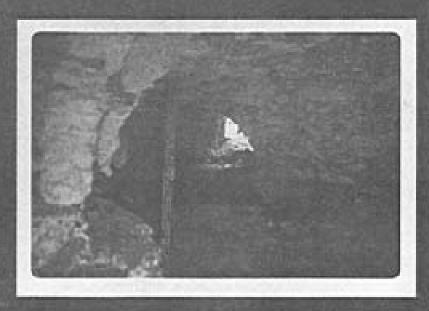
Photo 38 Str.50-73, robbery tunnel locking from the centerline to the outside, after removal of accumulated debris.
