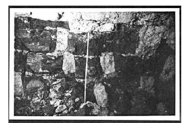
Photo 15 Bu. 196, upper courses of north wall with stretcher stones collapsed but butts of headers visible.
