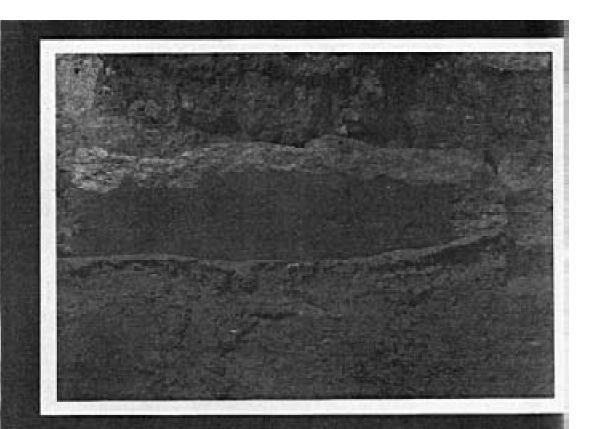
Photo 22 Bu. 196, south wall top showing where vault mortar was caught by the wall-top cover-cloth.
