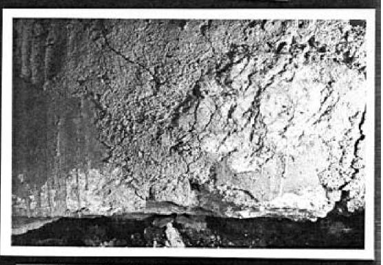
Fhoto 27 St. 196, drip lines of vault mortar (north side t).
