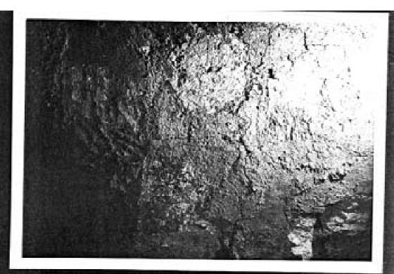
Photo 26 Su. 196, drip lines of wault mortar.
