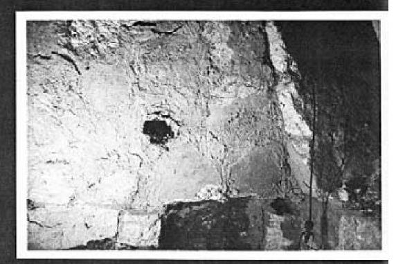
Photo 25 Bu. 196, finger marks in vault mortar (north vault).
