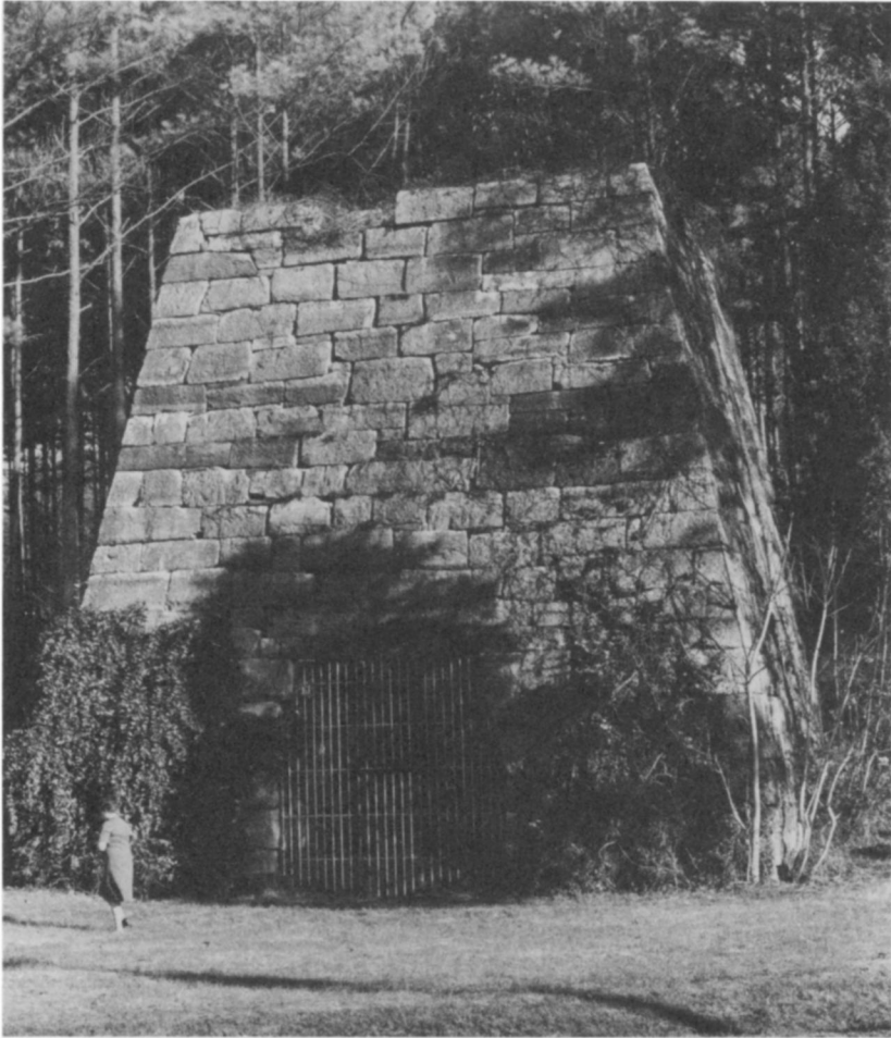
Fig. 2. Glenwood Furnace, Rockbridge County, Virginia, as it appears today. This stack, thirty-eight feet high, was erected in 1849 and is typical of the charcoal blast furnaces built and manned largely by slave labor in Virginia during the late antebellum decades. Photograph courtesy Mr. T. T. Brady, Richmond, Virginia.
