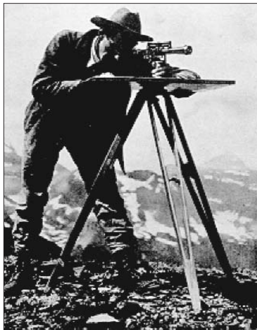
Surveying the scene. Early USGS mappers used plane tables and alidades to get the lay of the land.
