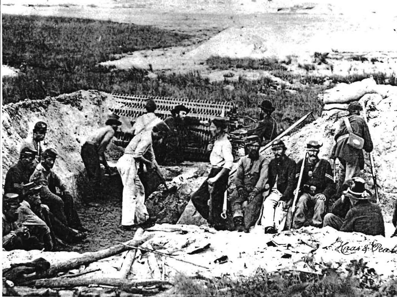
Engineers and men of the 54th working close to Fort Wagner behind a "sap roller."
