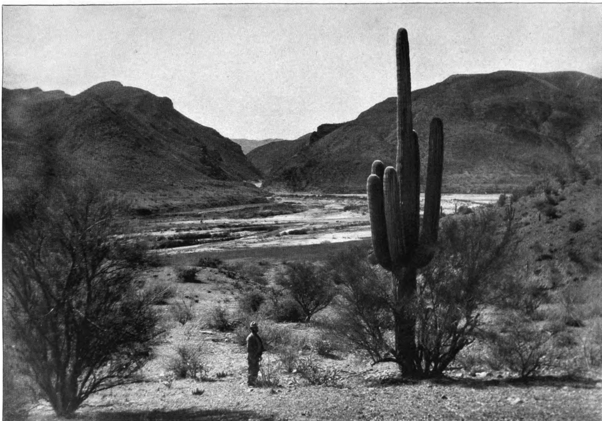
HUDSON RESERVOIR AND CANAL COMPANY'S DAM SITE IN THE DISTANCE.
