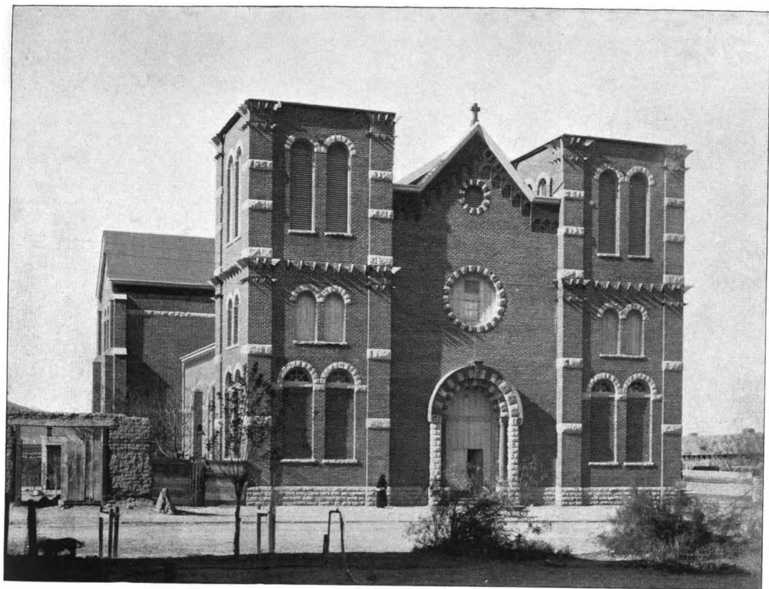
TUCSON CATHEDRAL, TUCSON.
