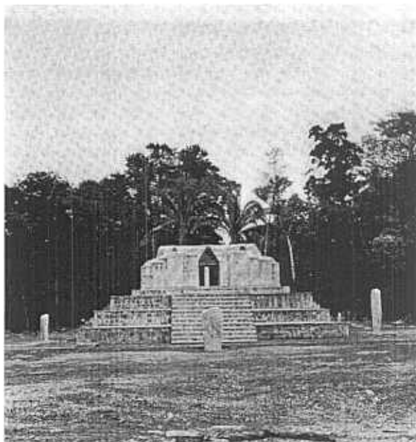
Fig. 7. — South side of Structure A-3 after reconstruction. Notice stela in central room.
