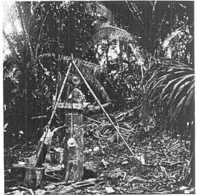
Fig. 19. — Putting the top part of Stela 2 in place.
