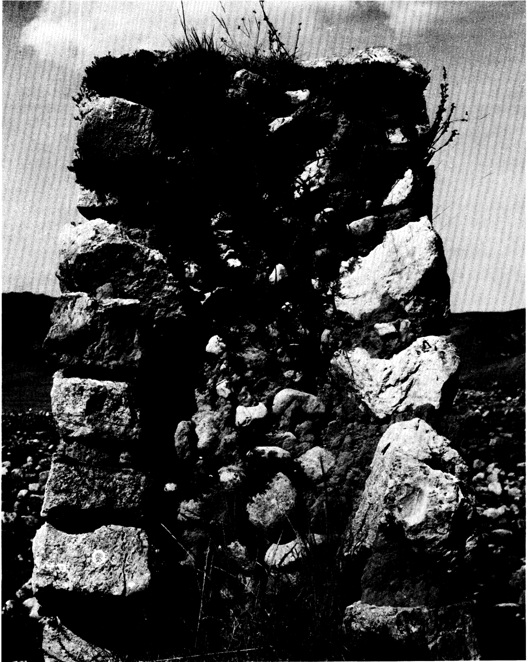
Fig. 8. Cross section of a house wall in the northern quarter of the city. Wall is of pirka masonry, bifacial with a rubble fill.
