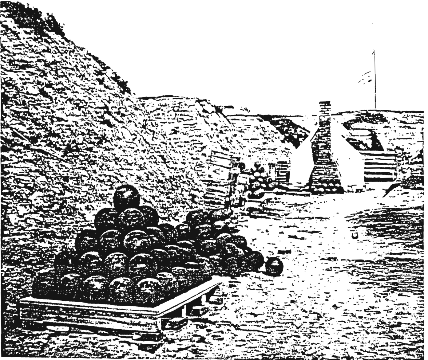
Above: Interior rear of the four-gun "water battery." Bomb-proof rear right under flag; guns are at left behind revetments.
