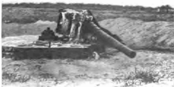
WEST BATTERY, CAVITÉ, AFTER DESTRUCTION
