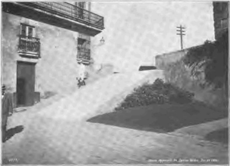
CORTINA DE VALDES. RAMP AT SOUTH END, DECEMBER, 1900.
