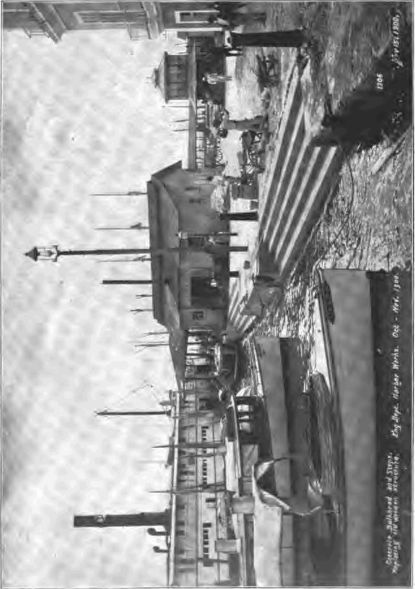
CONCRETE BULKHEAD AND STEPS, REPLACING OLD WOODEN STRUCTURE.
