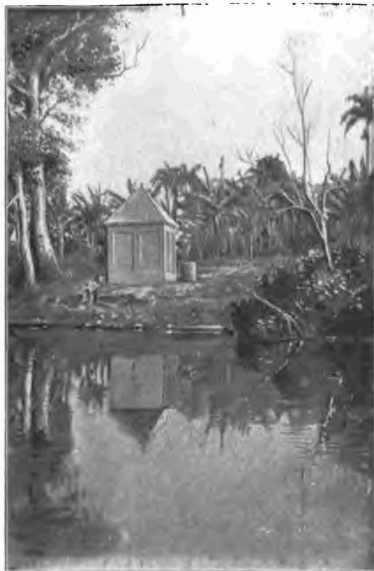
VALVE HOUSE NO. 2.
