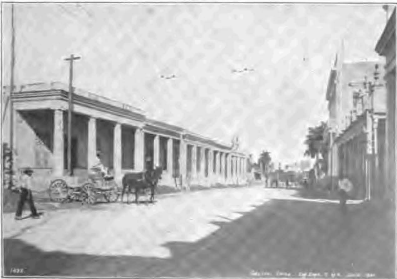
CALZADA DEL CERRO, AFTER NEW TRACKS WERE LAID, JANUARY, 1901.
