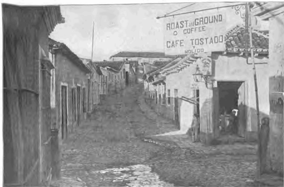
HOSPITAL STREET, NORTH FROM JAGUEY STREET, BEFORE IMPROVEMENT.
