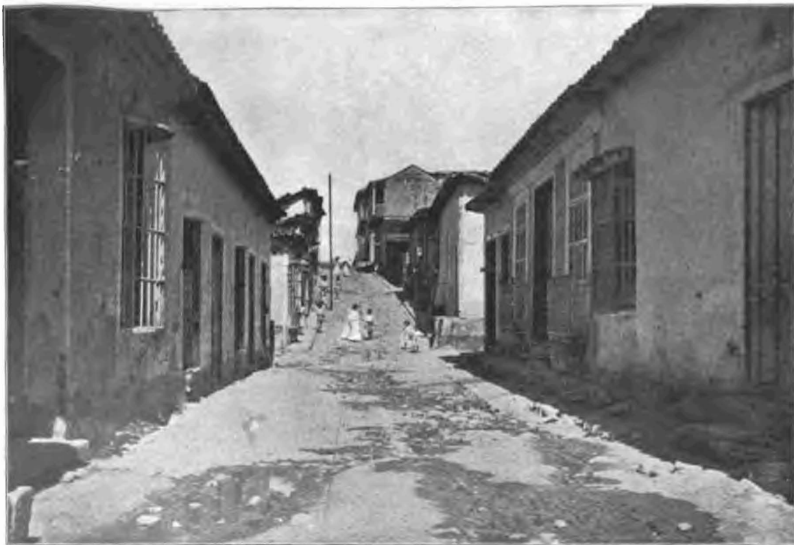
HOSPITAL STREET, SANTA LUCIA TO HEREDIA, BEFORE IMPROVEMENT.
