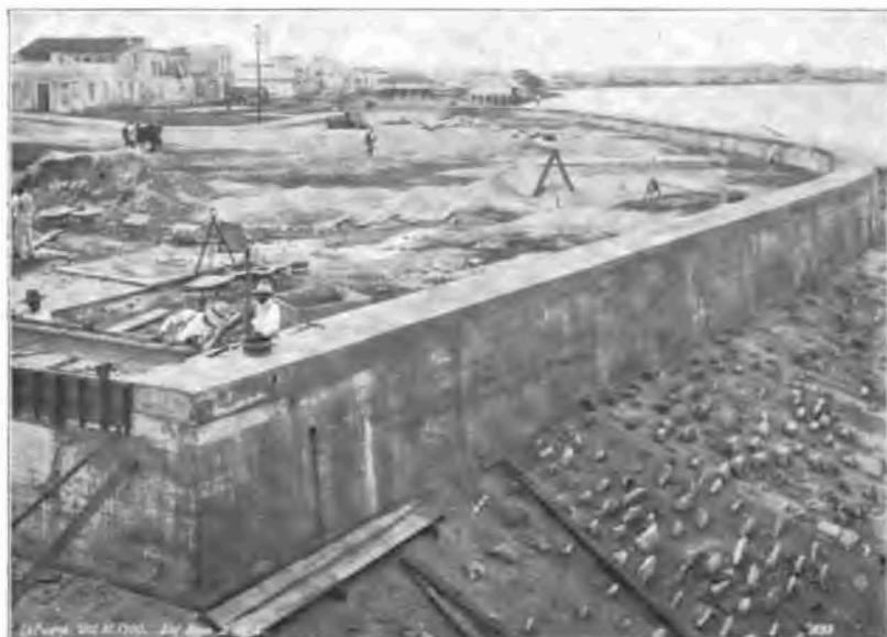
SEA WALL AT LA PUNTA. COPING MOSTLY COMPLETED, OCTOBER, 1900.
