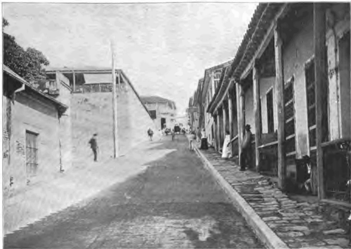
HEREDIA STREET, ANIMAS TO HOSPITAL. BRICK PAVEMENT COMPLETED.
