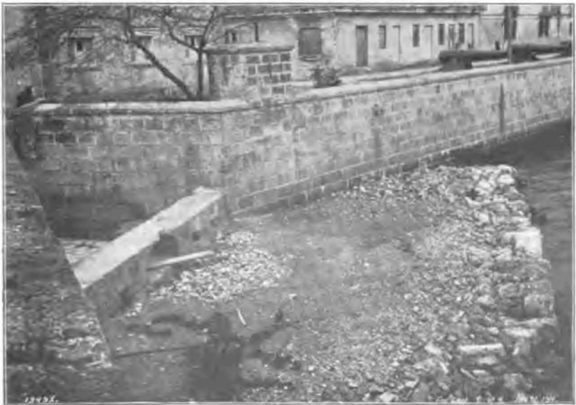
EXTENSION OF TACON STREET SEWER. FILLING IN PLACE, JANUARY, 1901.
