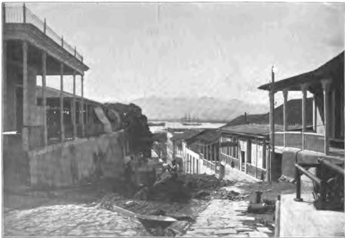
MARINA STREET HILL, SEWER WORK.
