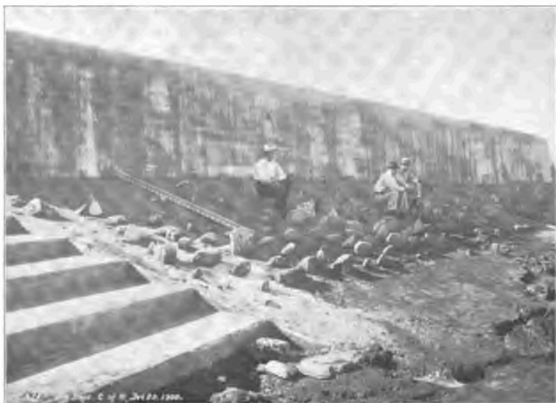
SEA WALL AT LA PUNTA, SHOWING CONSTRUCTION OF TOE.
