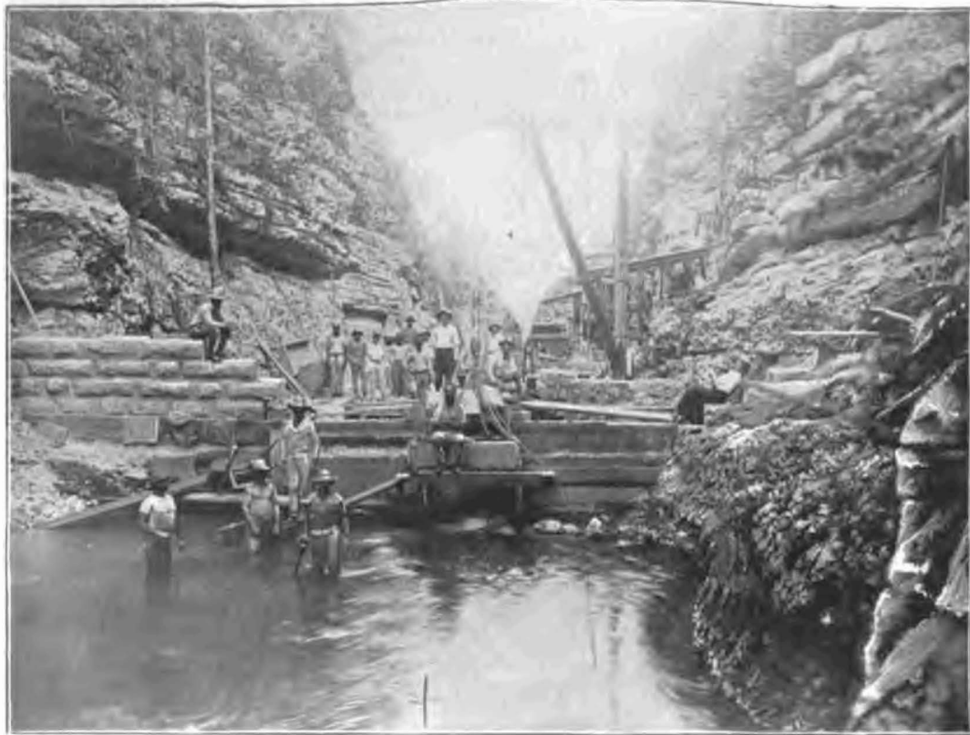
CLEARING RIVER BED ABOVE SLUICE.
