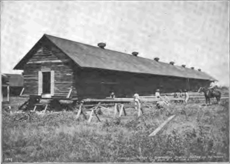
MOVING BUILDING TO QUARANTINE STATION. BLOCKED UP TO MOVE.
