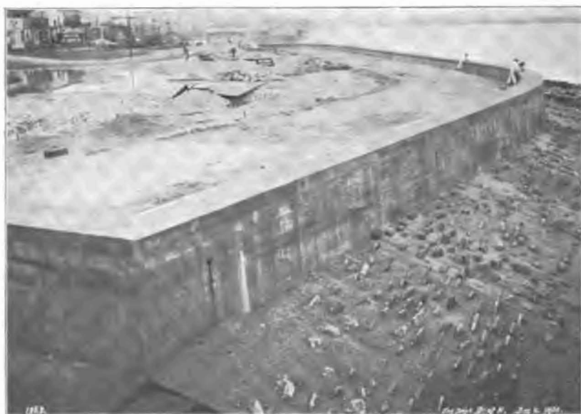
SEA WALL AT LA PUNTA. WALL COMPLETED, GRADING FINISHED, DECEMBER, 1900.
