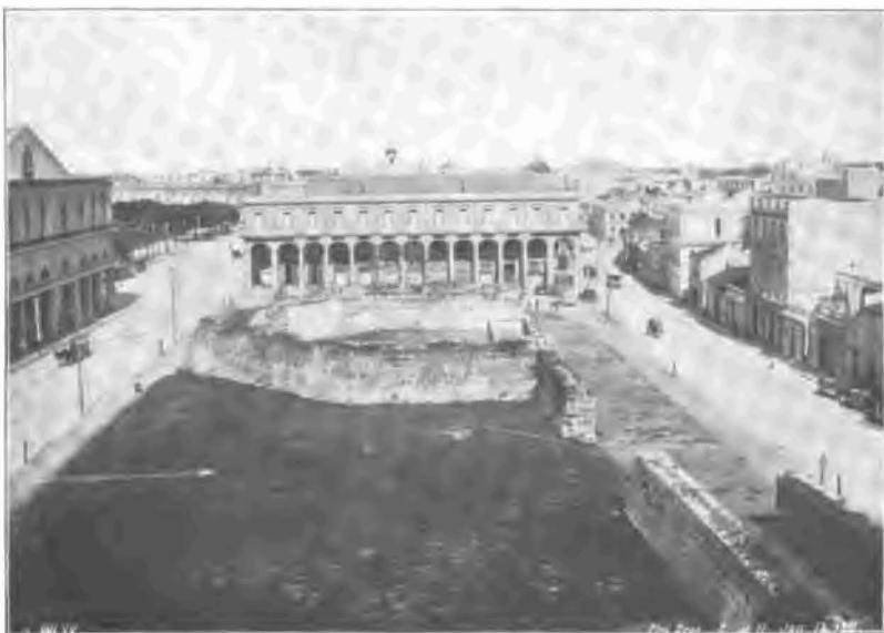
GRADING AND CLEANING LOTS AROUND PORTIONS OF OLD CITY WALL. NORTH LOT, JANUARY, 1901.
