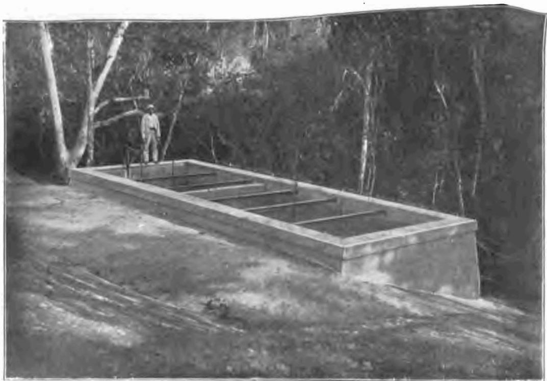
SAND BOX COMPLETE, EXCEPT PLANK COVER.
