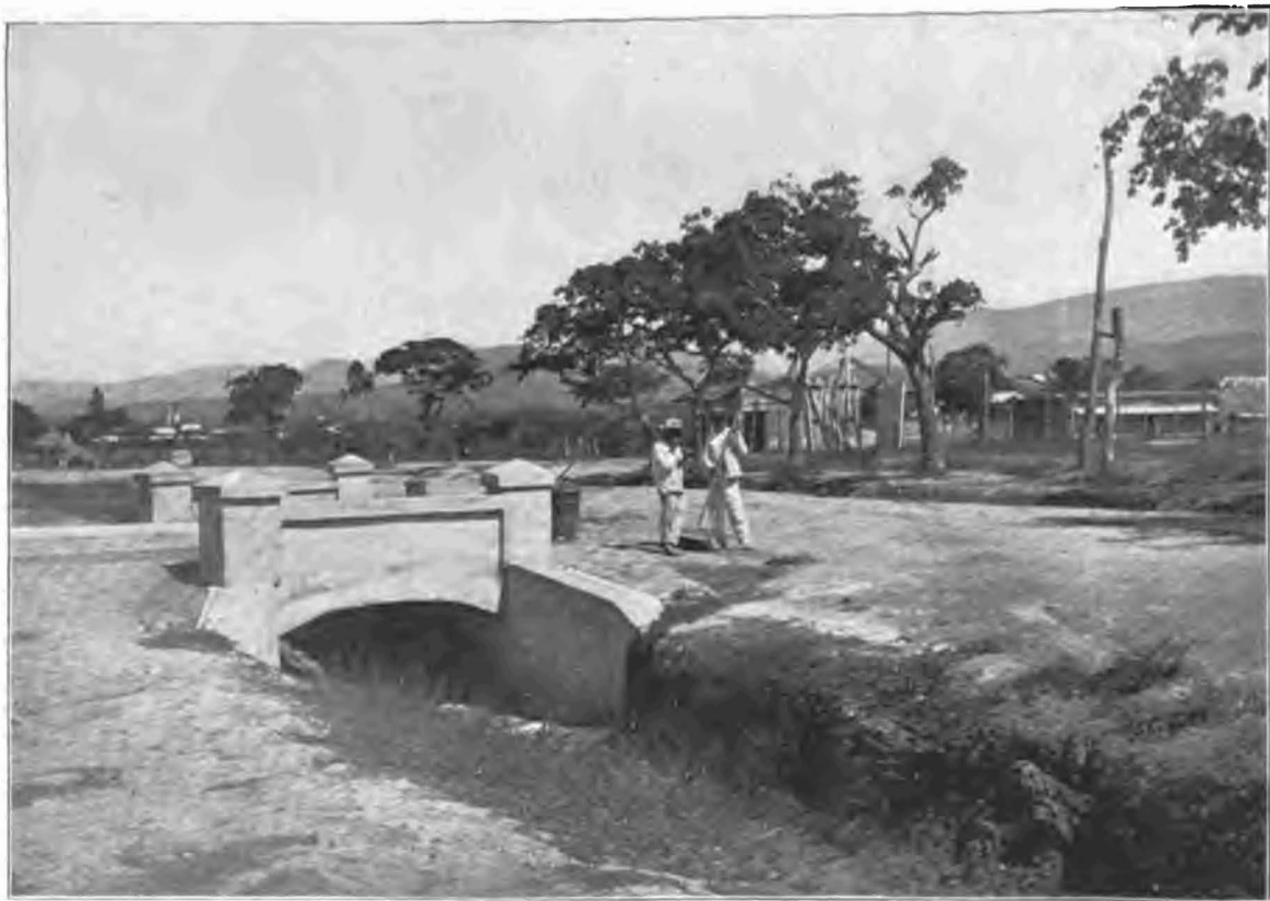
SAN FELIX STREET AND CONCHA ROAD. CULVERT.
