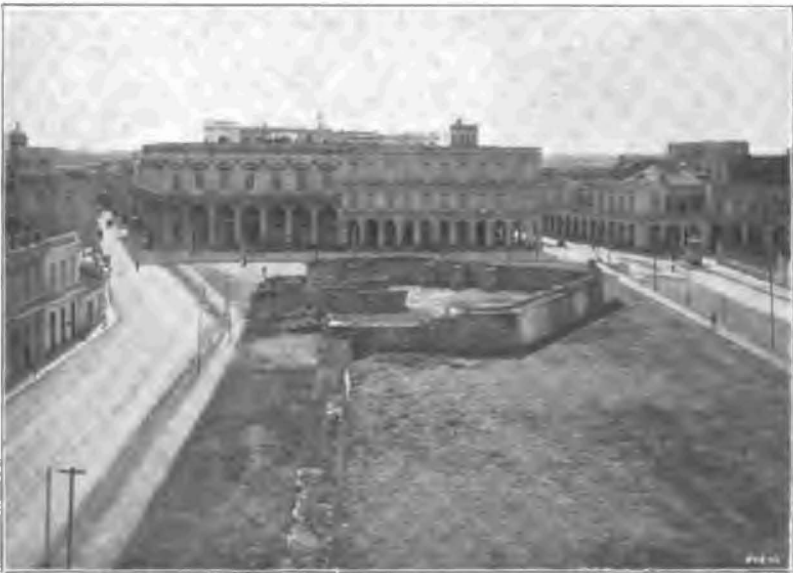
GRADING AND CLEANING LOTS AROUND PORTIONS OF OLD CITY WALL. SOUTH LOT, JANUARY, 1901.
