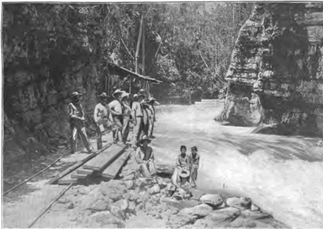
VIEW BELOW DAM. REBUILDING TRACK. WATER FLOWING 14 INCHES OVER DAM, SEPTEMBER 17, 1900.
