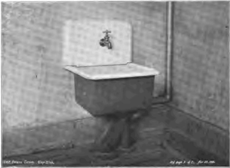
HABANA CARCEL. SLOP SINK.
