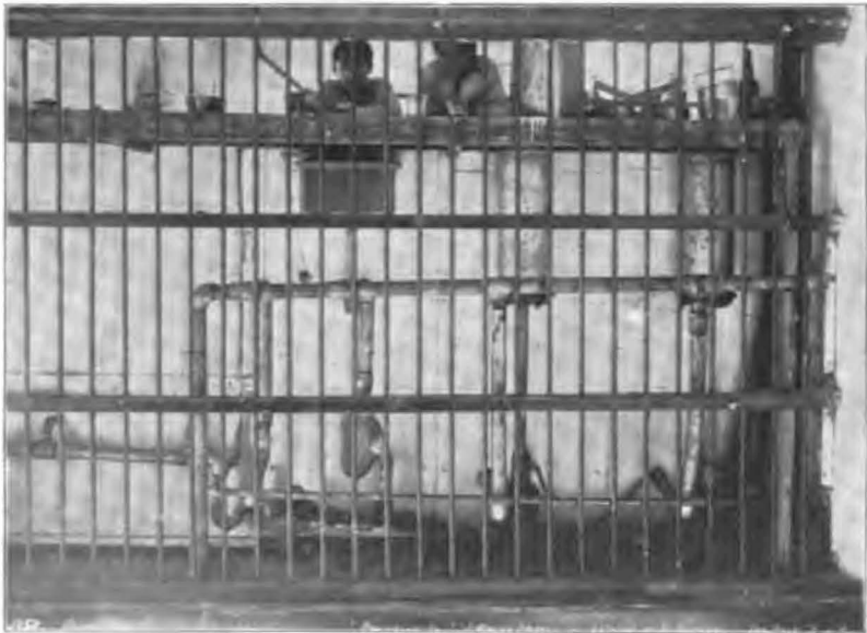
HABANA CARCEL. "ROUGHING IN" TWO WATER-CLOSETS, ONE URINAL, THREE BASINS.
