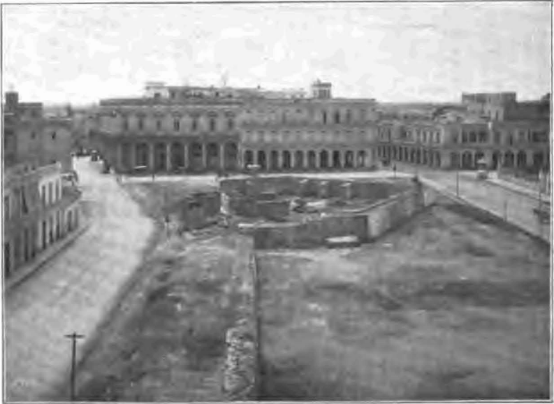
GRADING AND CLEANING LOTS AROUND PORTIONS OF OLD CITY WALL. SOUTH LOT, AUGUST, 1900.
