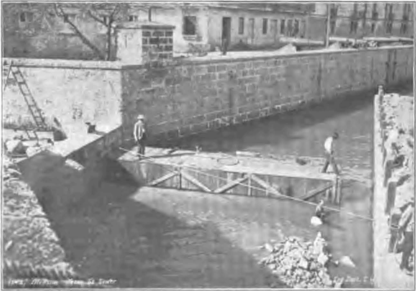
EXTENSION OF TACON STREET SEWER. BOX SEWER IN PLACE, NOVEMBER 1, 1900.
