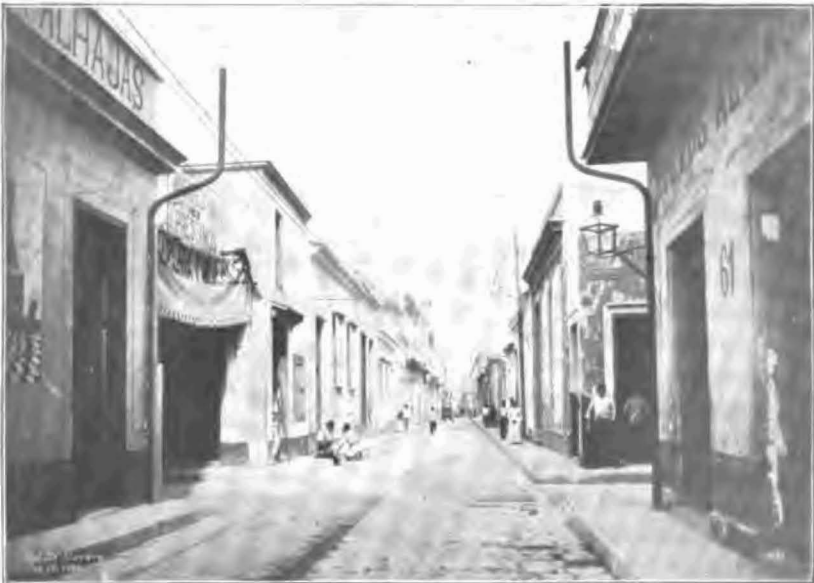
HABANA ELECTRIC RAILWAY COMPANY. POLE LOCATION ON NARROW STREETS; TRUSSES NOT YET IN POSITION.
