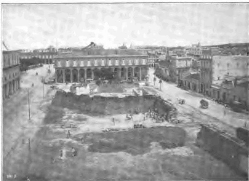
GRADING AND CLEANING LOTS AROUND PORTIONS OF OLD CITY WALL. NORTH LOT, AUGUST, 1900.
