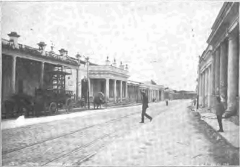
CALZADA DE JESUS DEL MONTE, AFTER NEW TRACKS WERE LAID, JANUARY 1, 1901.
