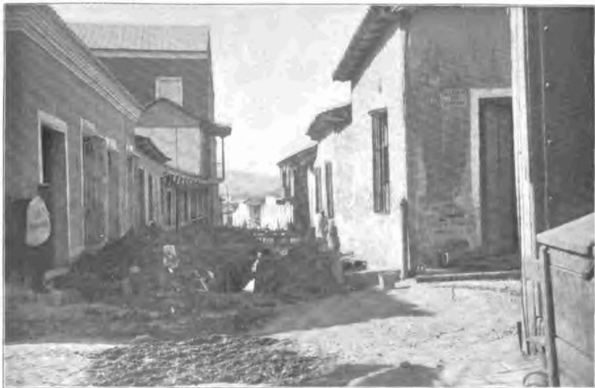
JAGUEY STREET, WEST FROM HOSPITAL. SEWER AND WATERWORKS.
