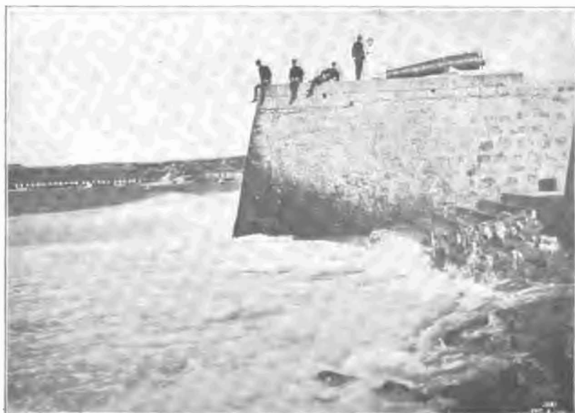
SEA WALL AT LA PUNTA. EFFECT OF TOE ON WAVE ACTION.
