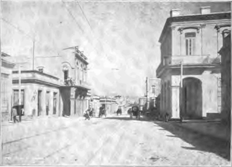
HABANA ELECTRIC RAILWAY COMPANY. POLE LOCATION ON WIDE STREETS.
