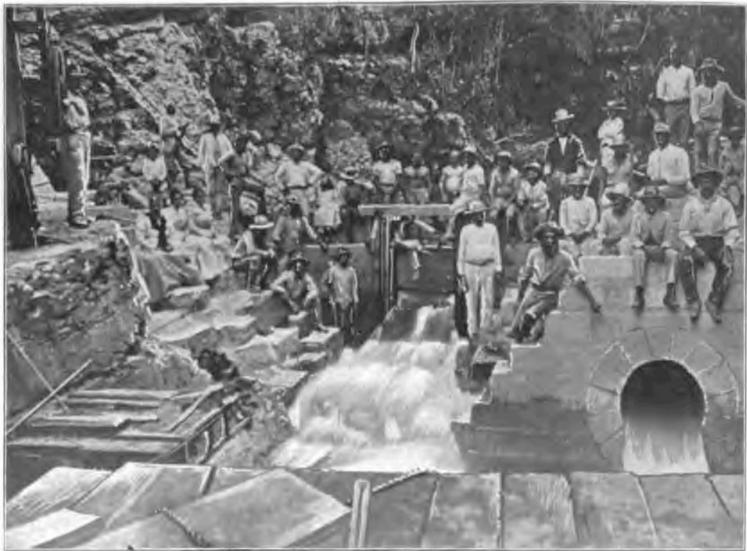
FLUME REMOVED. PLACING COFFERDAM, AUGUST 27, 1900.
