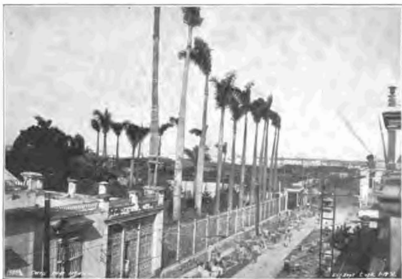
TRACK LAYING, HABANA ELECTRIC RAILWAY COMPANY, CALZADA DEL CERRO.
