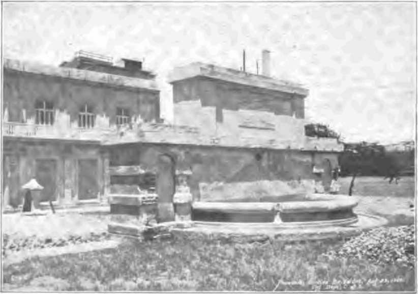
CORTINA DE VALDES. FOUNTAIN AT NORTH END, AUGUST, 1900.
