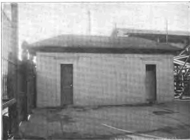
HABANA MATADERO. TOILET ROOM.
