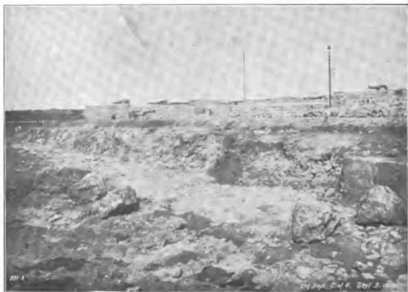
SEA WALL AT LA PUNTA. EXCAVATING, SEPTEMBER, 1900.
