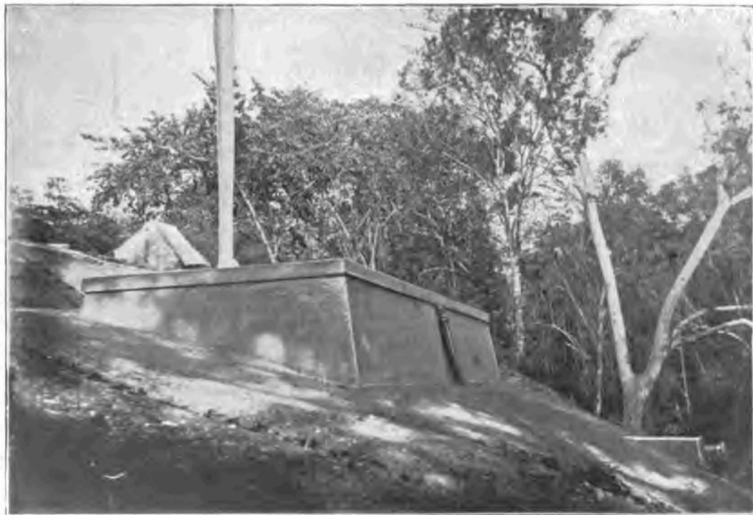
SAND BOX, LOWER SIDE, SHOWING OVERFLOW PIPE.
