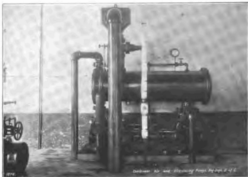
CONDENSER, AIR AND CIRCULATING PUMPS.
