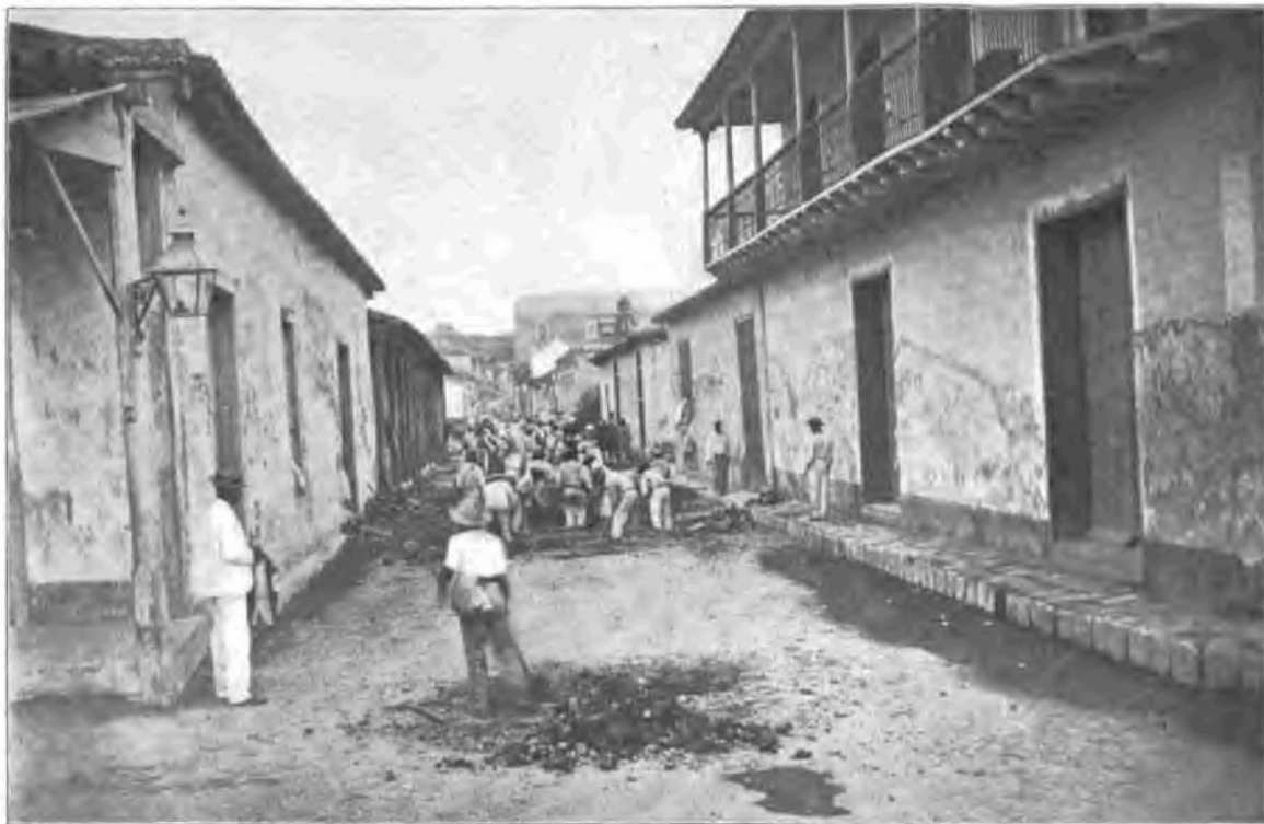
JAGUEY STREET, CHRISTINA EAST. WORK ON SEWER.
