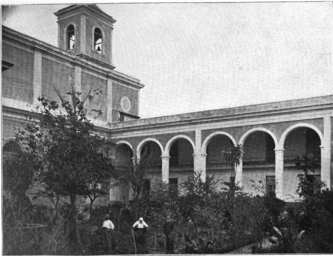
SAN LAZARO LEPER HOSPITAL, HABANA, CUBA. PATIO, WOMEN'S SIDE.
