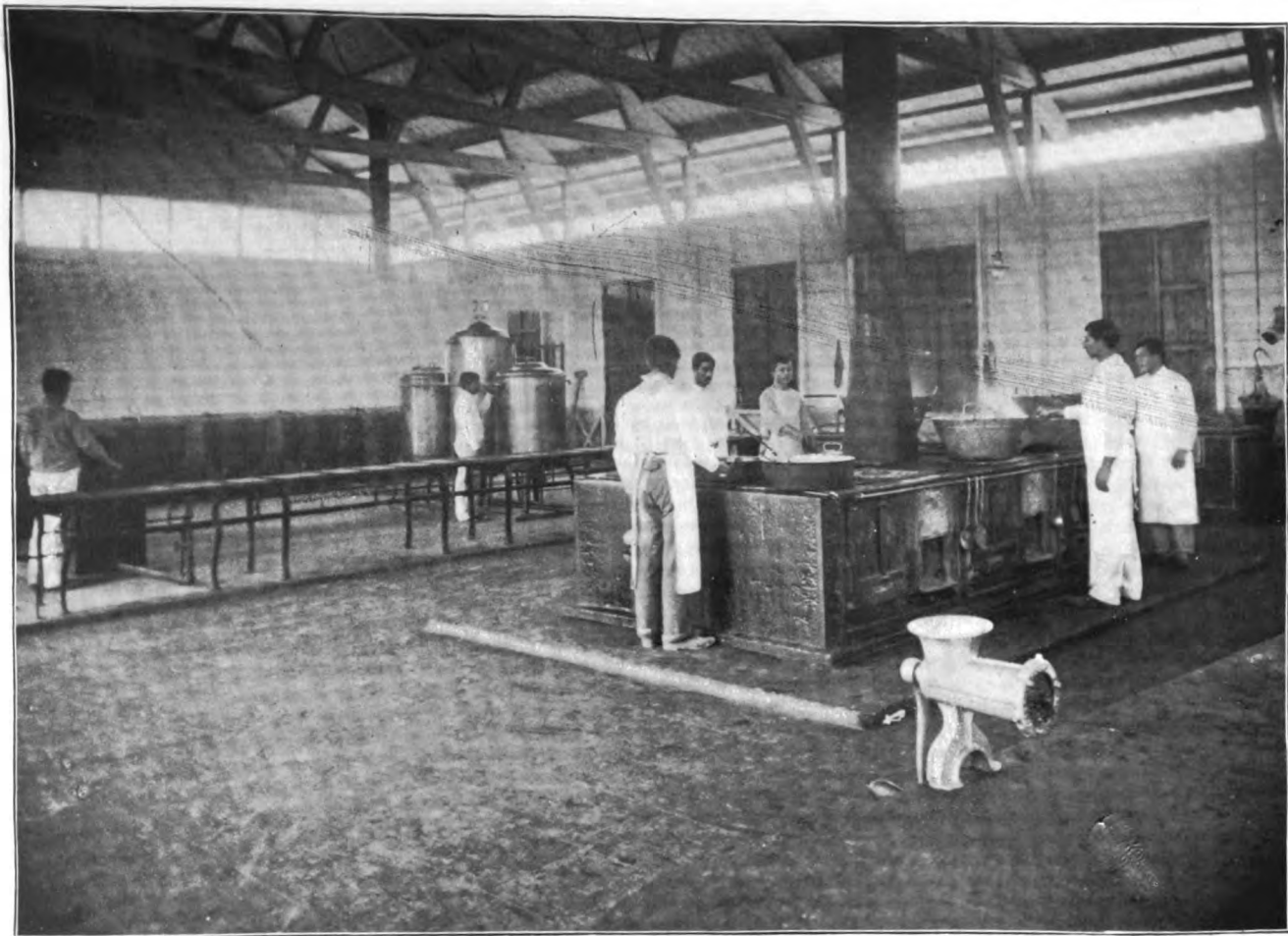
MUNICIPAL HOSPITAL NO. 1, HABANA, CUBA. KITCHEN.
