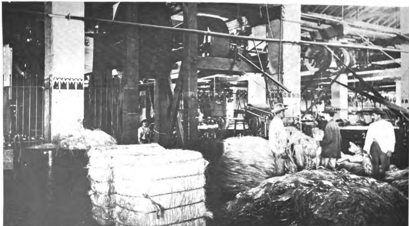
CORDAGE FACTORY OF HEYDRICH, RAFFLOER & CO., HABANA. PREPARATION DEPARTMENT NO. 1.
