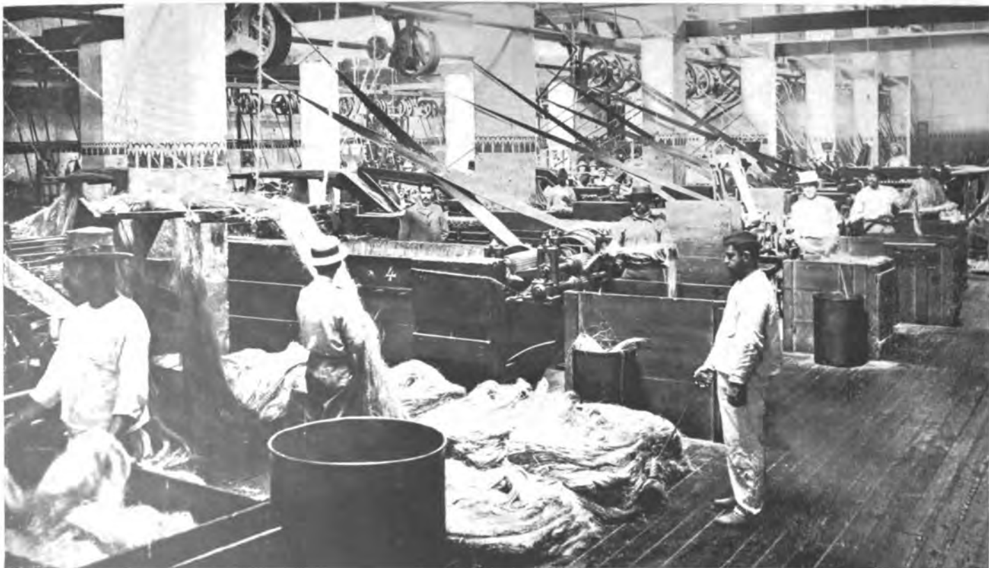
CORDAGE FACTORY OF HEYDRICH, RAFFLOER & CO., HABANA. PREPARATION DEPARTMENT NO. 2.
