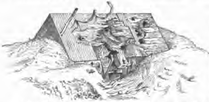
CASEMATE ON THE EASTERN CURTAIN OF FORT HINDMAN, SHOWING THE EFFECT OF SHOT FROM THE UNION GUNS.
